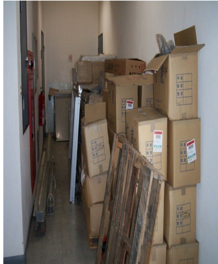
Emergency exit obstructed by materials
