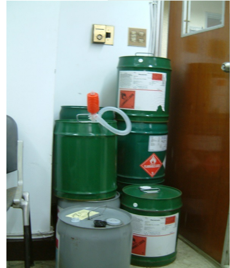
Emergency door obstructed by chemicals
