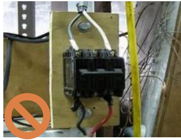
Unsafe electric facility
